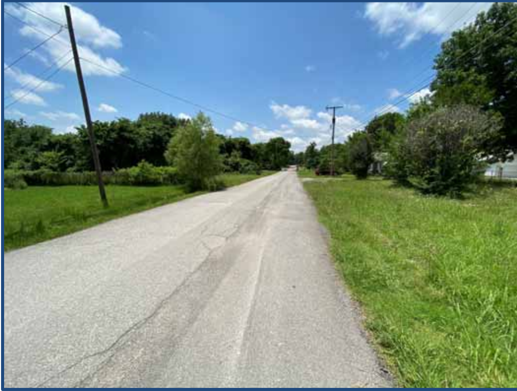
View West on East Jackson Street – Subject on Right
